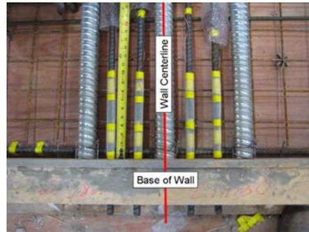
Figure 7. Placement and Unbonded Length of Mild Steel Bars Crossing Base Joint
